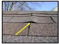
• **Repair:** There should be no exposed nail heads through any flashing material, shingles, capping or vent boots on roofs. Such nail heads will rust and cause a leak. There are exposed nail heads at several locations which should be covered with roofing cement or other sealant to prevent them from rusting and causing a potential leak. This is not generally an expensive repair.
