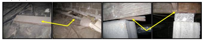
• **Improve:** Termite shields are required to be installed at the top of the foundation block under the framing members and at the tops of all columns. Termite shields are installed to help prevent termites from reaching the framing members of the house. There were no termite shields installed in the crawlspace of the home. It is recommended that termite shields be properly installed.
