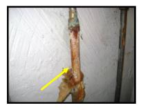
• **Repair:** The hose bibs (exterior faucets) are not properly secured to the building. The collar should be securely fastened into the brick or substrate by a mechanical means.
