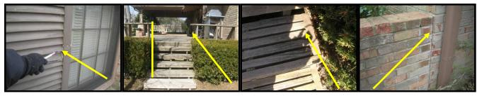
**Improve:** All shrubs and vegetation should be cut back away from the building at least 12 -24" to promote proper air circulation around the walls. Vines and other climbing plants can cause damage to exterior surfaces and should not be allowed to grow on the building. Such vegetation also prevents proper drying of the siding and provides a pathway for insect life which can cause damage to your home.
