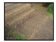
• Repair: There are some settlement cracks in the cement of the garage floor apron. It is recommended that they be filled to prevent moisture from entering and eroding the surface beneath the cement which will lead to additional cracking. Sonneborn and Trimco make some excellent long lasting products to help seal such cracks. Exterior Materials, 665 Wedgewood Ave. Nashville, TN (near the State Fair Grounds) carries Sonneborn and Trimco products.
