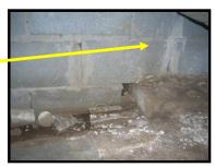
• Repair: Possible moisture intrusion was observed at the base of the inside corners of the garage. It is suspected that surface water is infiltrating these areas. Addressing the lot and gutter drainage should help to correct the condition. (See roofing section)
