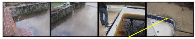
**Repair:** Deteriorated mortar joints and displacement was observed in the brick banding of the back patio. It is recommended that the damaged or missing bricks be repaired and all deteriorated mortar joints filled to prevent moisture intrusion. Some of the brick banding may have to be replaced to repair the displacement.
