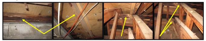
Repair: Localized wood rot was observed in much of the decking and some of the rafters of the pool pump house roof. It is recommended that the roof structure of the pool pump house be properly repaired.
