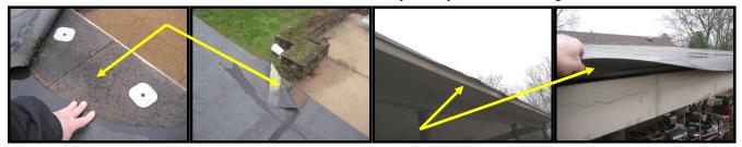
**Repair:** No gutters have been installed on the home. Properly installed gutters and downspouts will direct water away from the house and foundation which will help to maintain a dry crawl space or basement.
