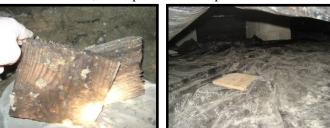
• **Improve: Information:** Some additional supports have been added in the crawl space of the house. The supports do not appear to have been installed in a workman like manor and it is recommended that they be improved.
